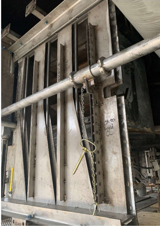
Figure 8: Birwelco USA Burner Compensator sliding plate, thrust bar, and removable pin (wind break removed).
