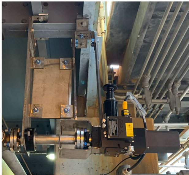
Figure 7: REXA Electraulic linear actuator driving Birwelco USA Burner Compensator assembly thrust bar.
