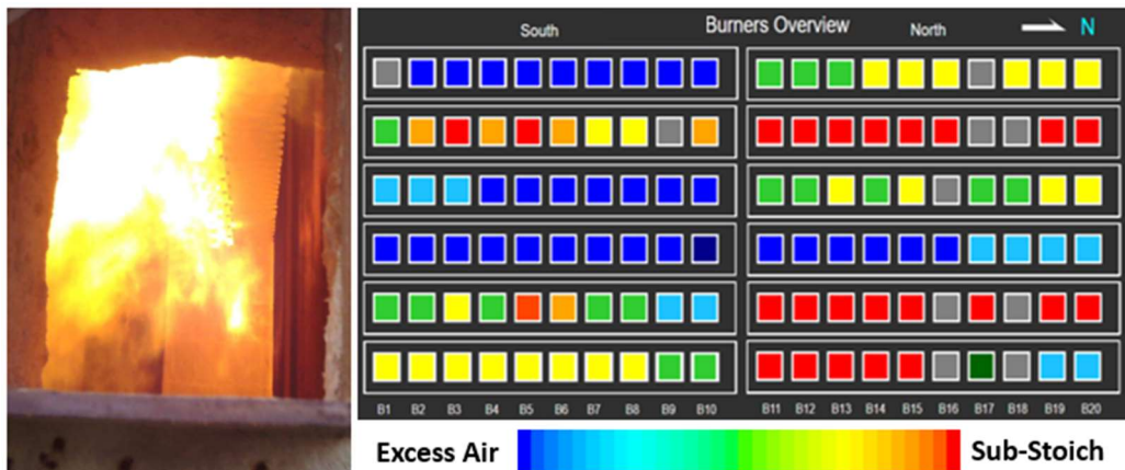
Figure 1: Excess air map - Mal-distribution induced by un-optimized tuning.
