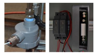
Figure 6 ClearSign EYE electronic modules: (Left) An electronic module (not visible) within a NEMA 4 rated enclosure connects to the probe and sends a 6-wire cable bundle out through conduit to the controller, (Right) the controller located in or nearby the burner management system panel.
