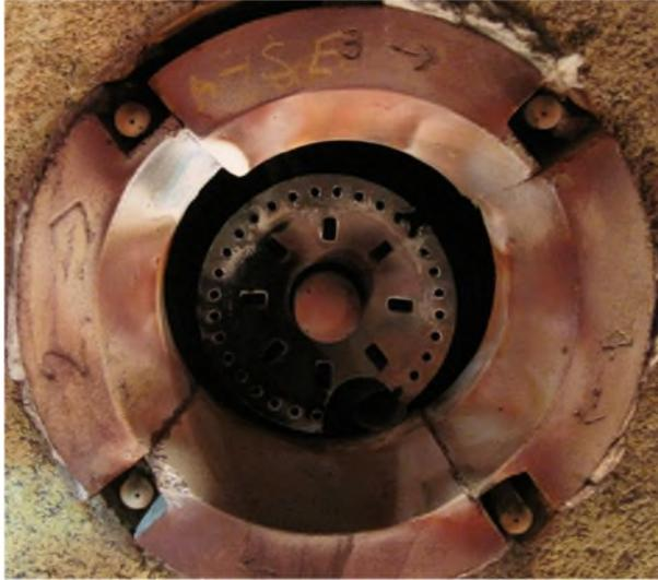
Figure 15 Burner tile segments improperly aligned.
