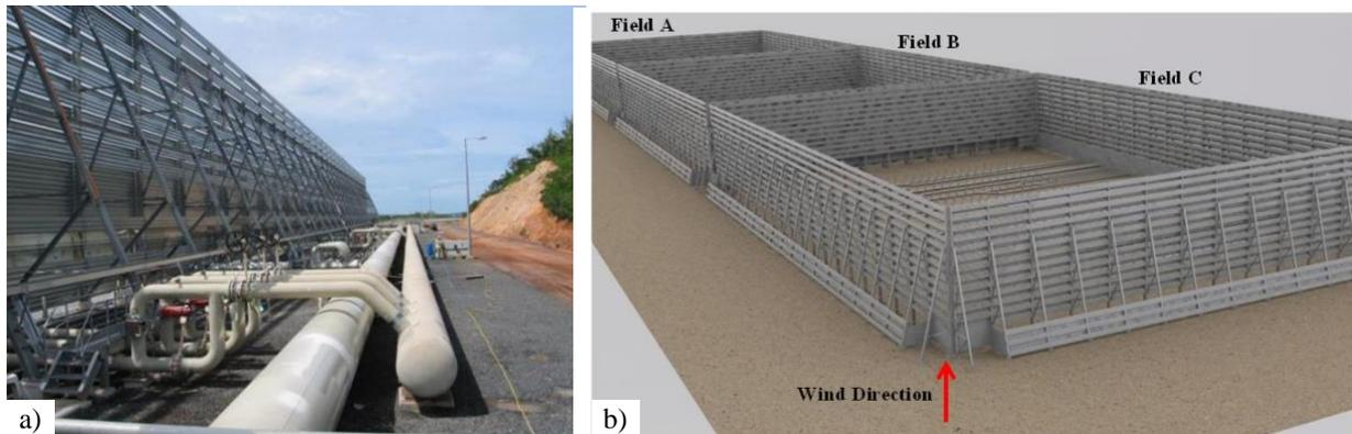
**Figure 9 - Large MPGF with: a) staging header and b) a surrounding wind fence for a multi-field flare system**
