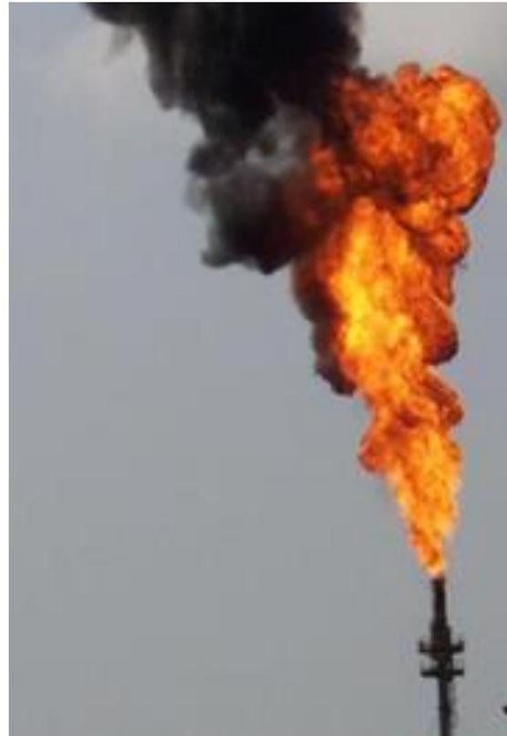
*Figure 1 – Flare flame moments after ignition showing black carbon emissions formed during transient ignition*
