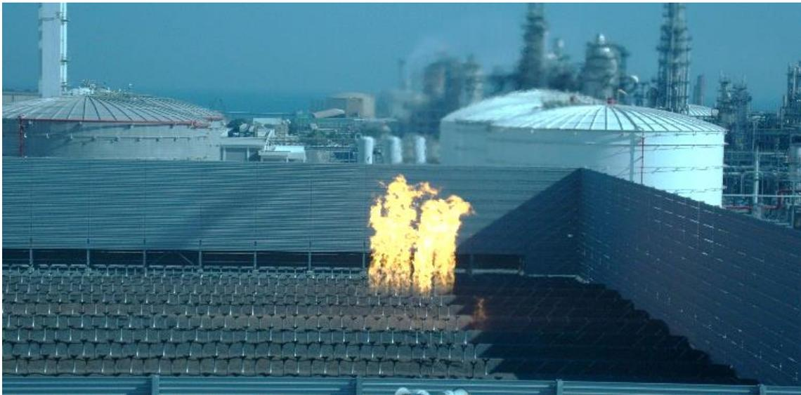
*Figure 2 - Multi-point ground flare contains hundreds of burners*
