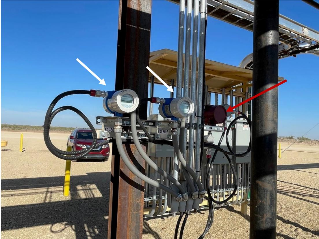
Figure 6. DRE-Max Automatic VFD Controller (Red Arrow) with Two Flow Meters (White Arrow) Used in Tests on July 27<sup>th</sup> 2022.
