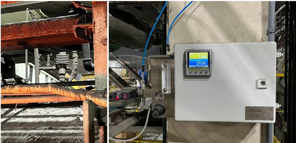
Figure 17. Oxysensor™ installation at copper furnace. Left: Probe. Right: Oxysensor™ cabinet/unit.
