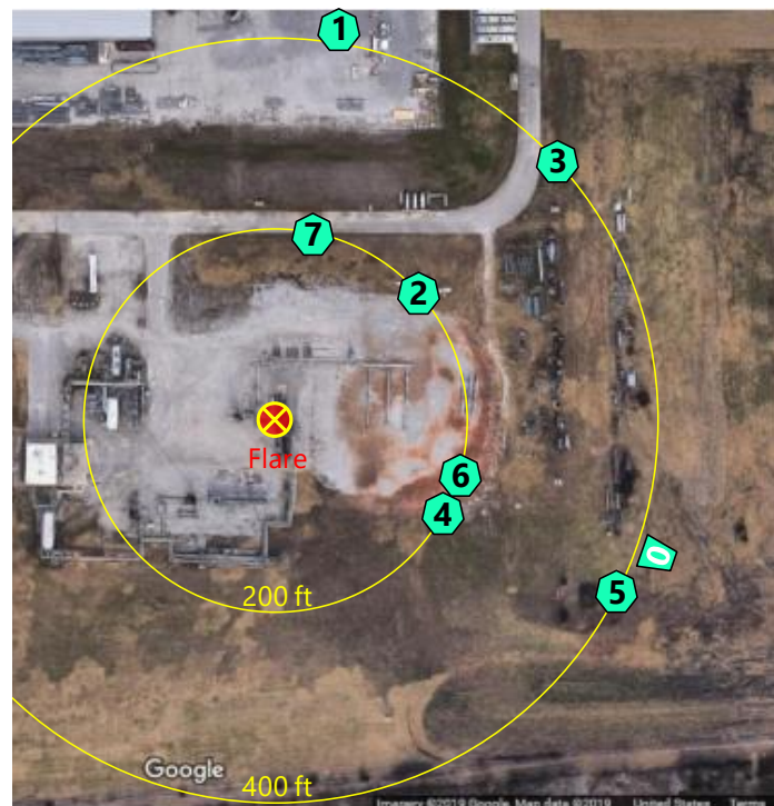
Figure 3: Site map showing the locations of the flare and the VISR devices during additional flare flow rate tests.
